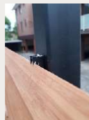
Aluminium strips screwed into the posts
