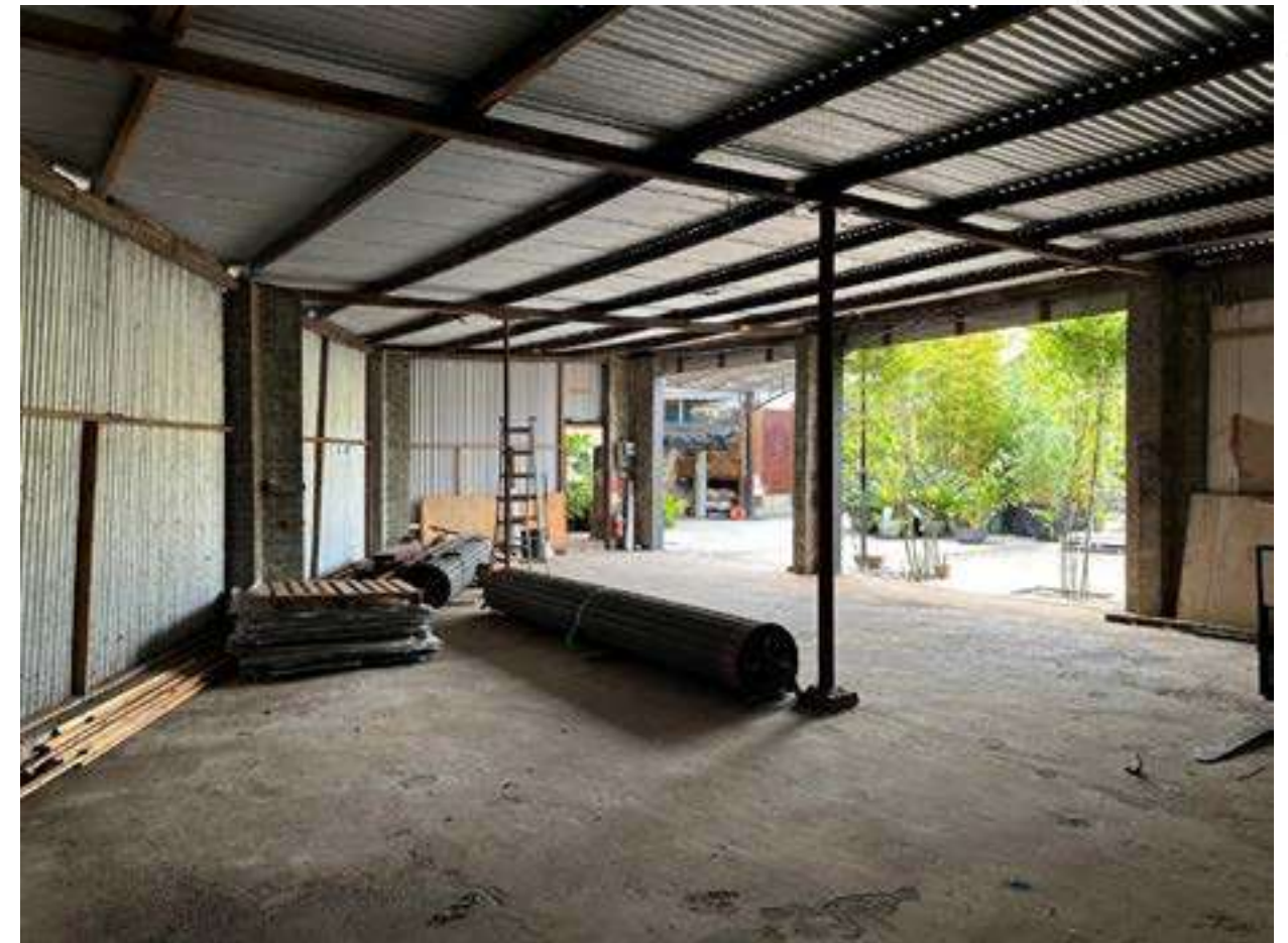
Existing storage space with roller shutters already removed.
