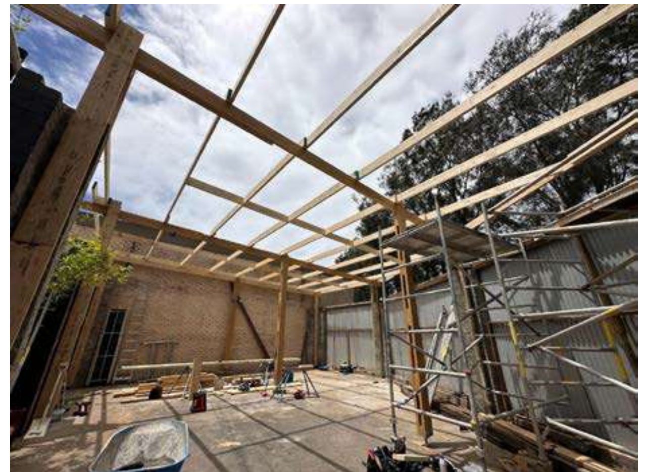
New engineered bamboo posts and roof structure in place
